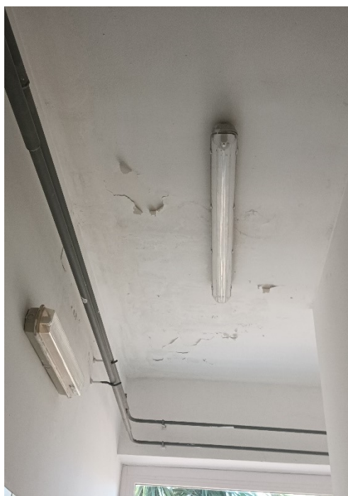
Bagno alunne piano terra pad. B
